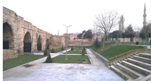
Figure 20. Relation with aqueduct
