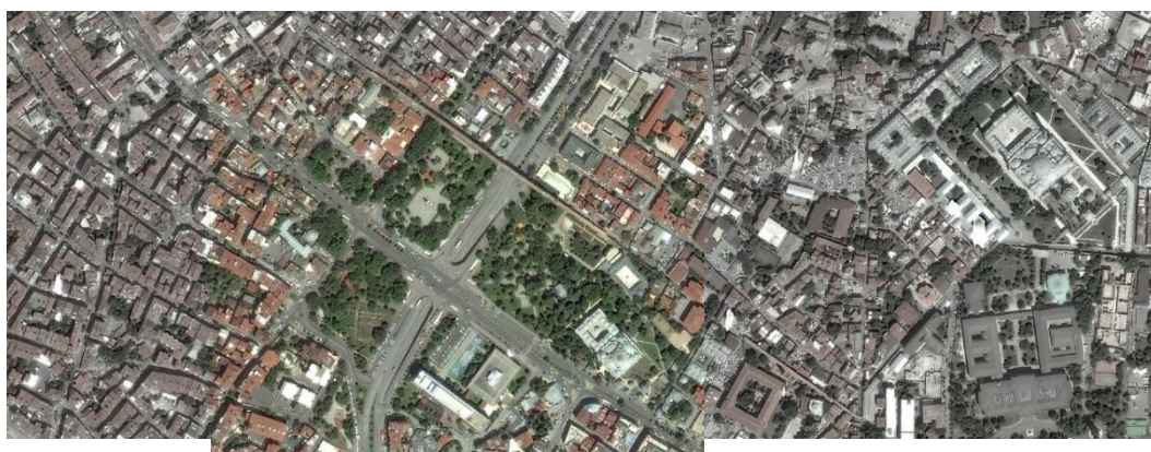
Figure 10. General view (source: Yandex Maps)
