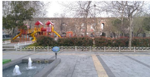
Figure 18. Children's Playgrounds and Aqueduct
