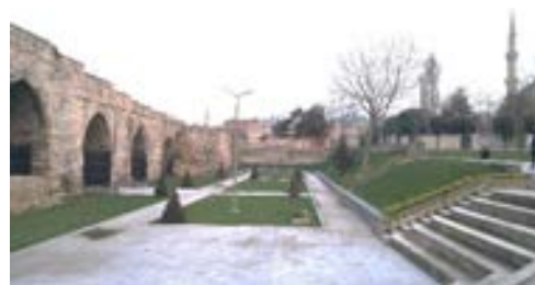
Figure 20. Relation with aqueduct
