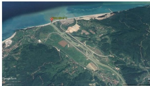
Figure 25. Filyos downstream satellite image (Google Earth, 2017)
