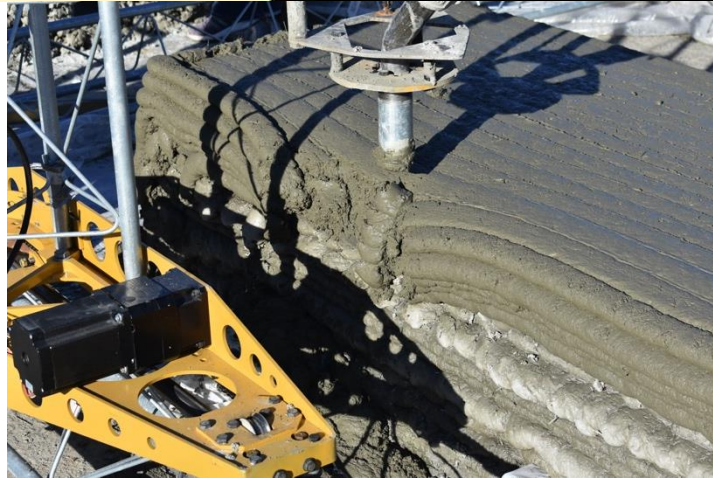
Figure 13. Material collapse under self-weight
