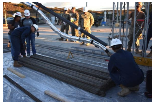
(b) Placing rebar on beam 1
